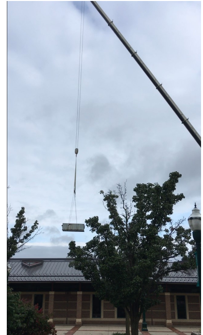
Old HVAC unit being removed from the library roof
